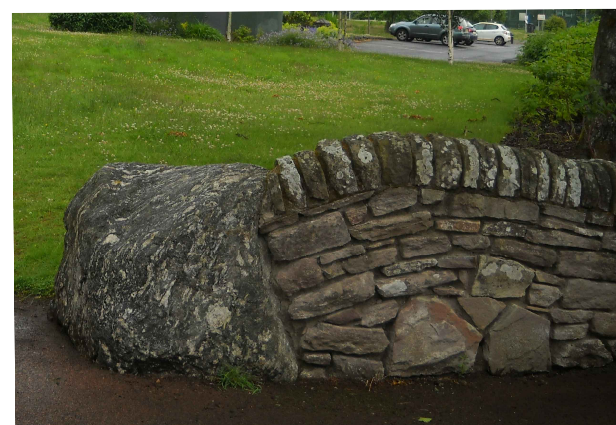
Above: Example of stone wall showing sandstone panel infill laid to courses, cope, glacial boulder end stone and recessed mortared joints. The workmanship for the proposed walls at the Knock shall match or exceed the quality of this wall which is located at the entrance to Larghan Park in Coupar Angus PH13 9AN
